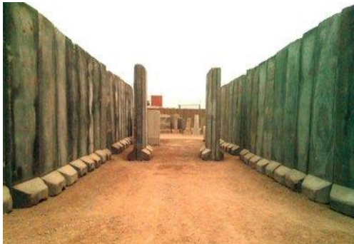
TYPE3. Outer protective wall ( T type concrete)
